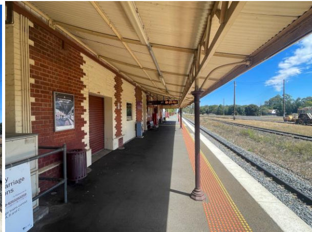
Detail of the platform area
