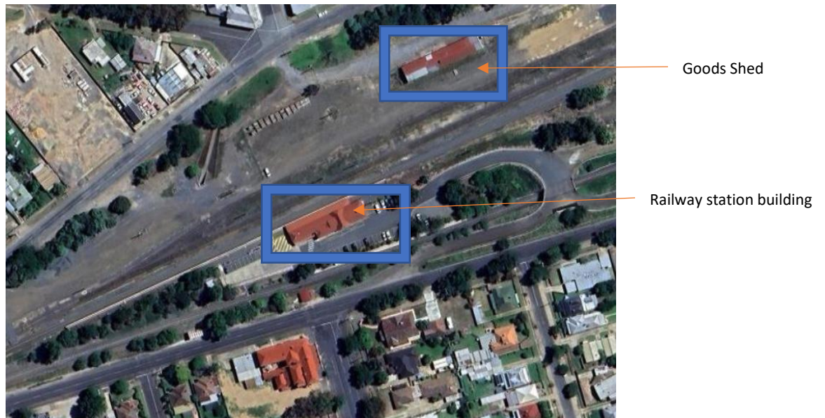
Aerial view of the station building and the approached
