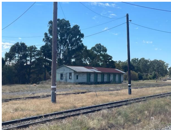
View to the Goods Shed (not included in any statement of significance)
