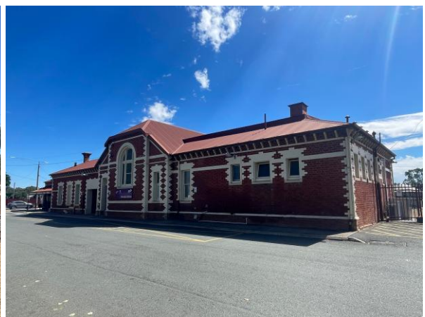
View to the station building from the car park area
