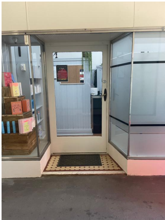
Typical original shop front
