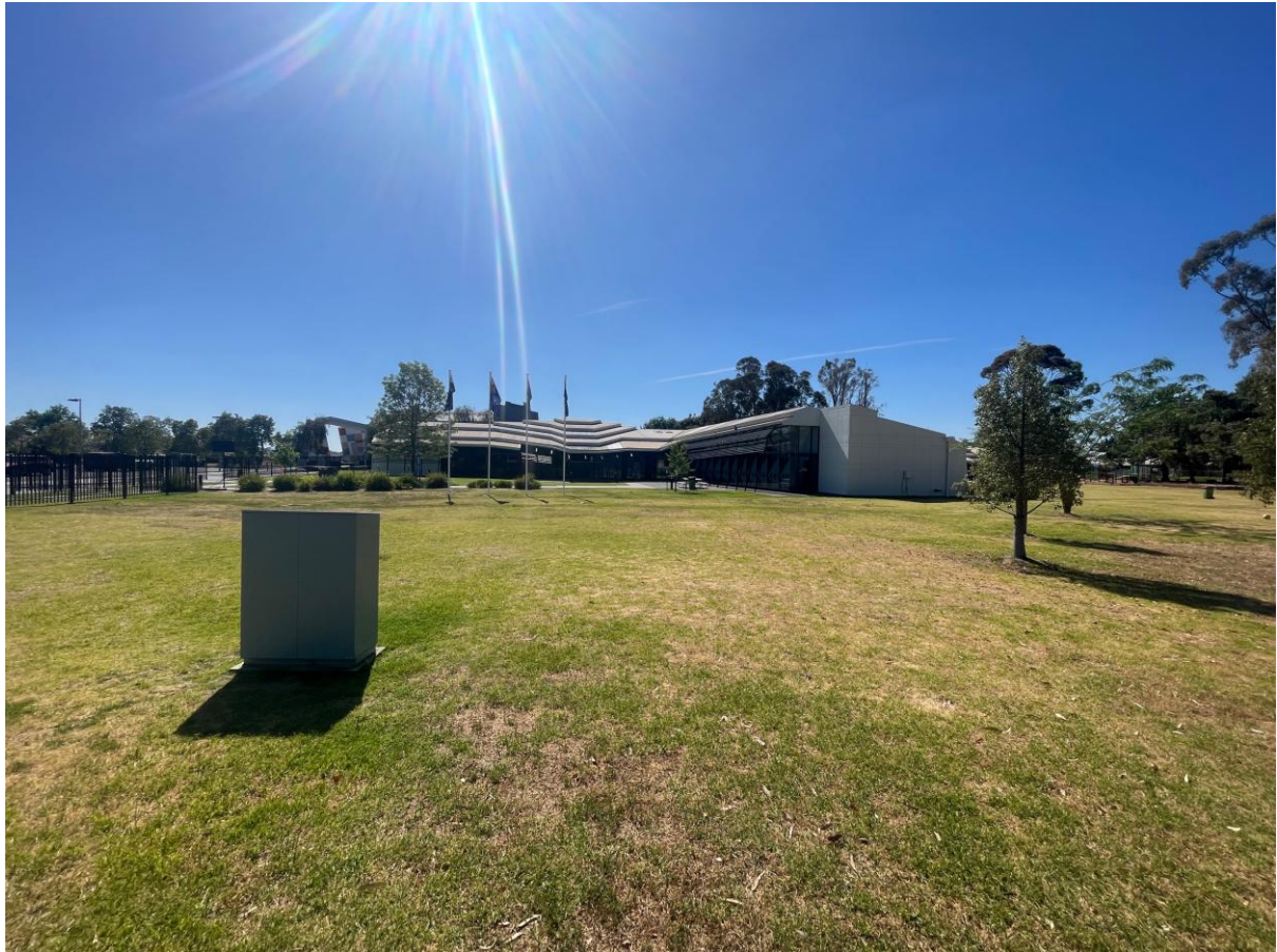
View to the building
