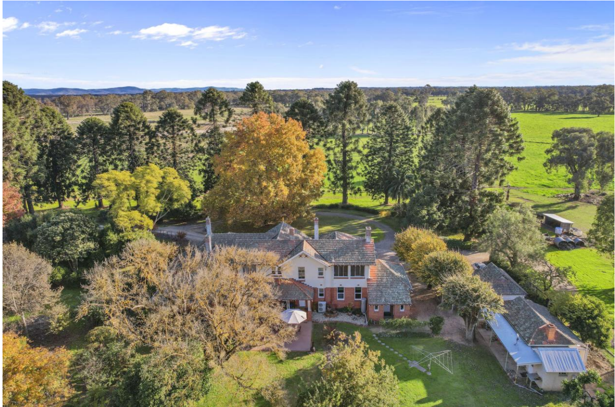
Figure 3 The Homestead constructed in the 1920s aerial perspective looking west (Source: LAWD)
