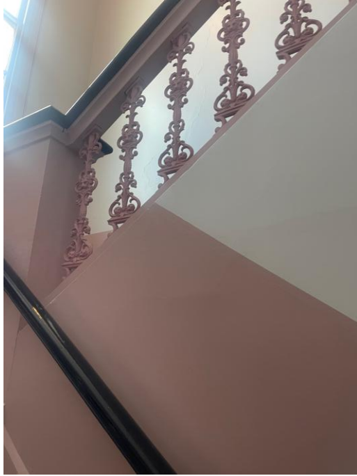
Detail of balusters
