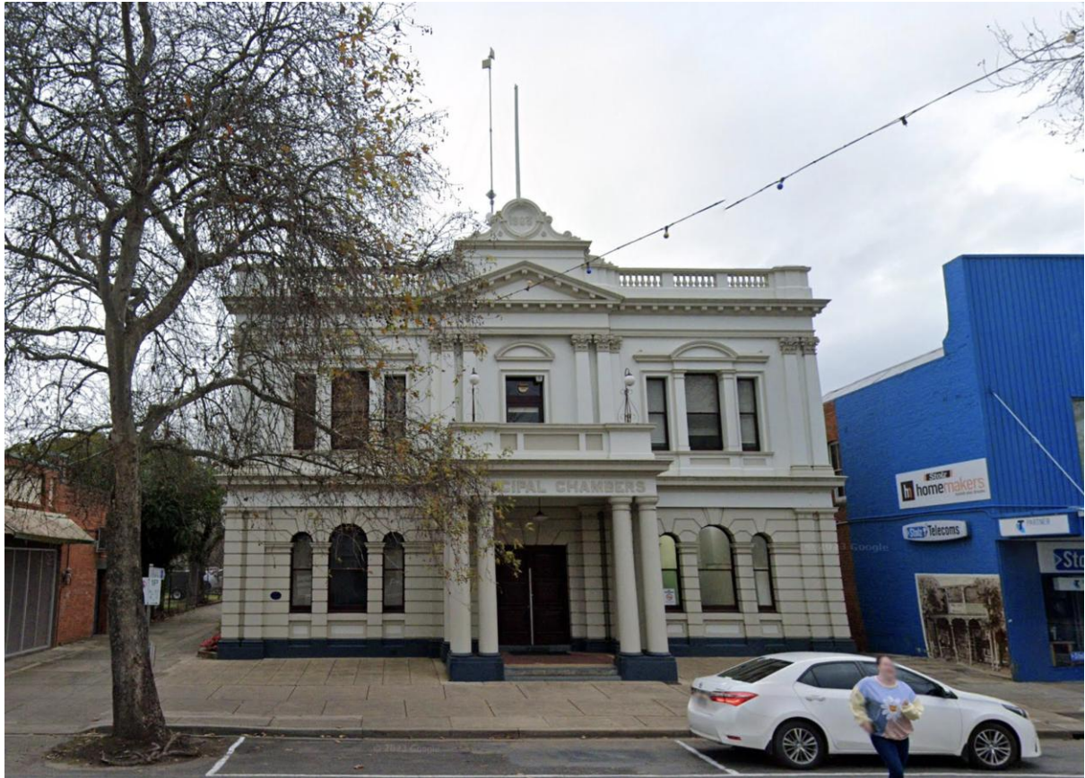
Benalla Shire Hall 82 – 86 Nunn Street Benalla
