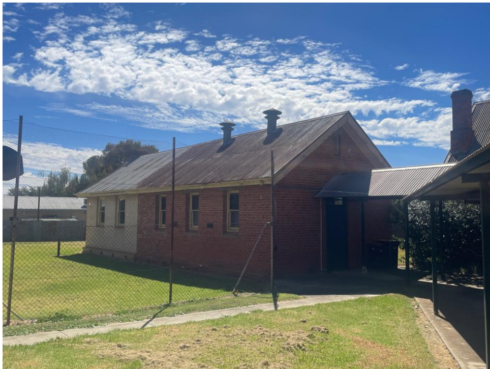
View to the hall to the rear of the church
